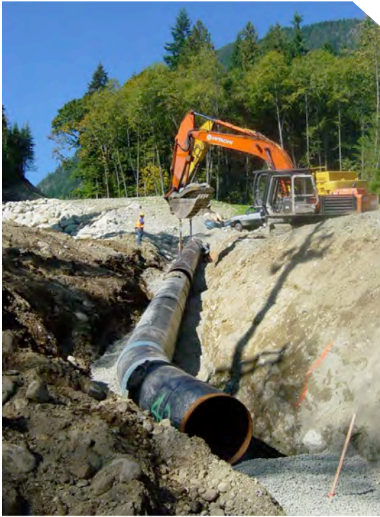
Installation of Penstock at McNair Creek Hydroelectric Project
