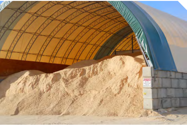
A biomass storage facility. Woody biomass sources in the province include existing mill wood residues, roadside debris and pine beetle damaged trees. The total generation potential for all wood sources is in the order of 2,300 MW.
