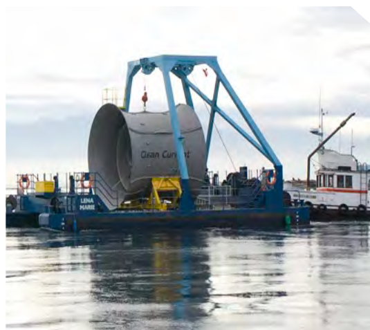
A tidal energy turbine being installed at Race Rocks.
